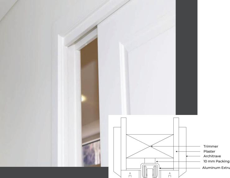
Aluminum Extrusion KD Hardware 13 mm - 21 mm
